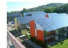
Fig 6: Use of photovoltaics on roofs in Freiburg, Germany (Alex Eby: CABE)
